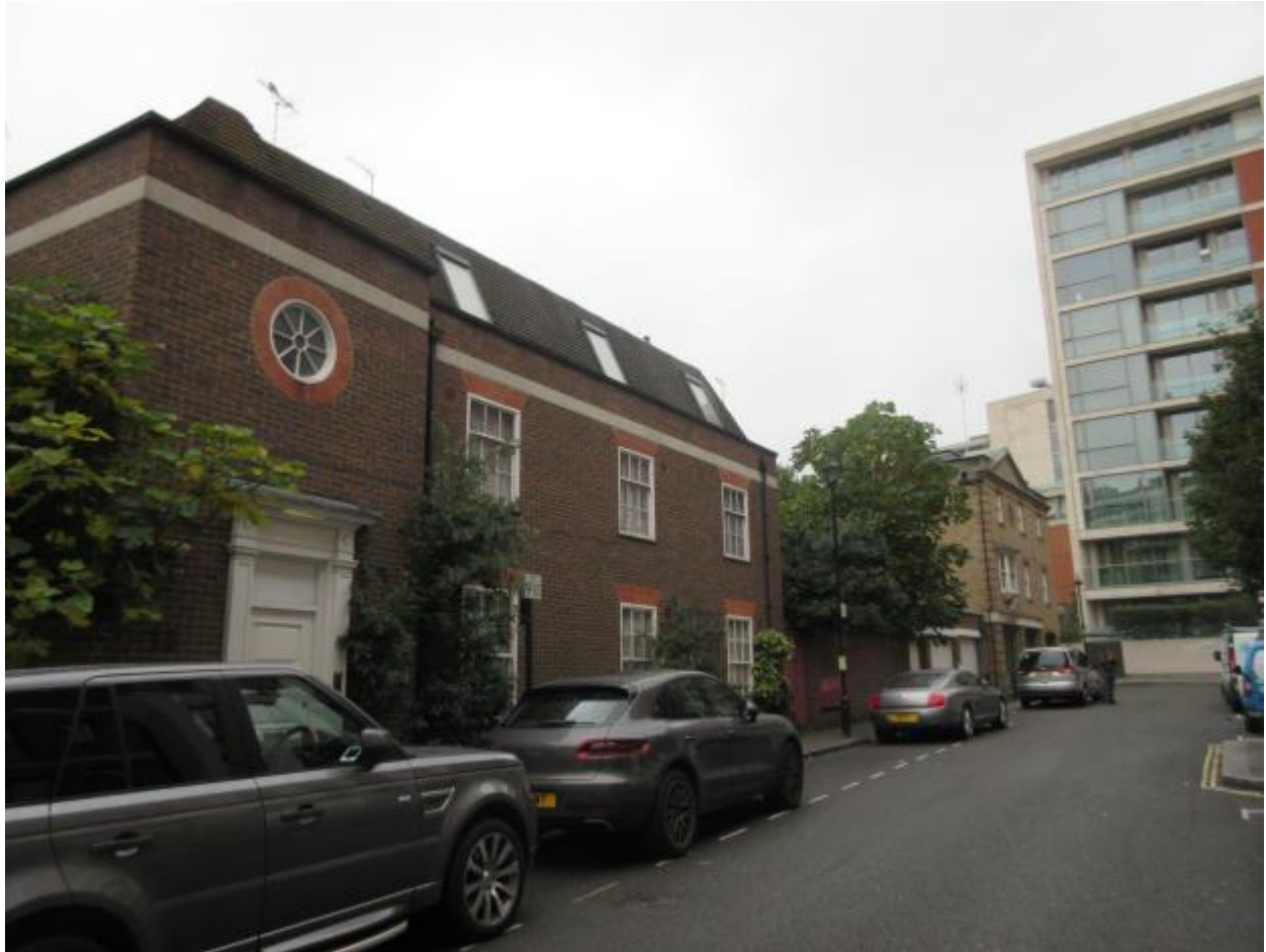
Front elevation of application site (15 Lancelot Place in the forefront and 1 Trevor Walk to the rear)
